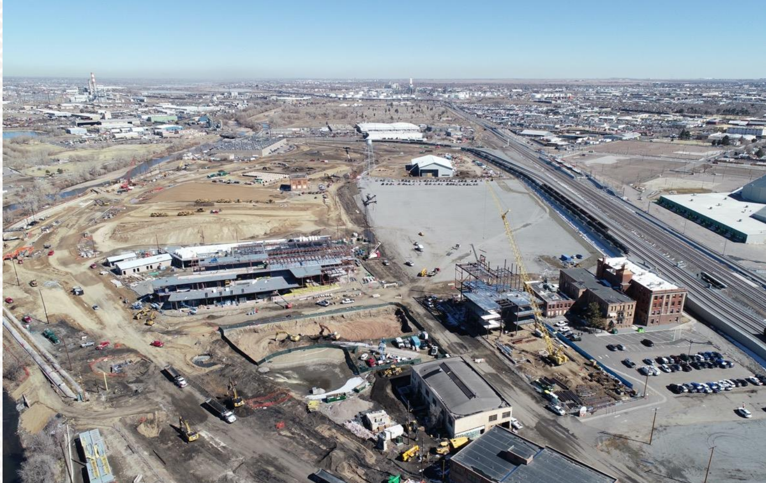
Sitework continues on the southern end of campus with the construction of Pond H – a permanent storm water detention pond.
